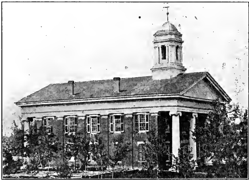
OLD COURT HOUSE
